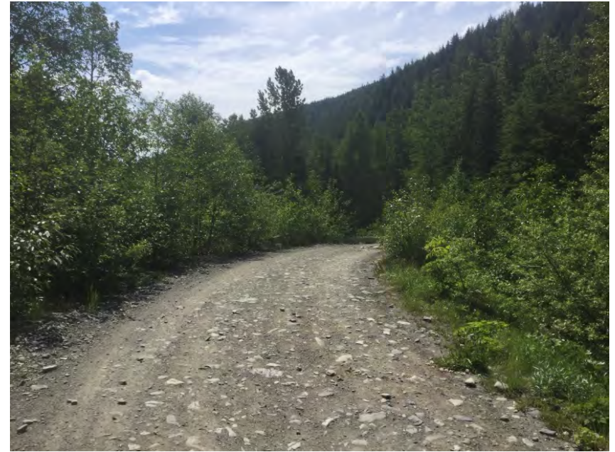
Approach from Left Bank when facing downstream
