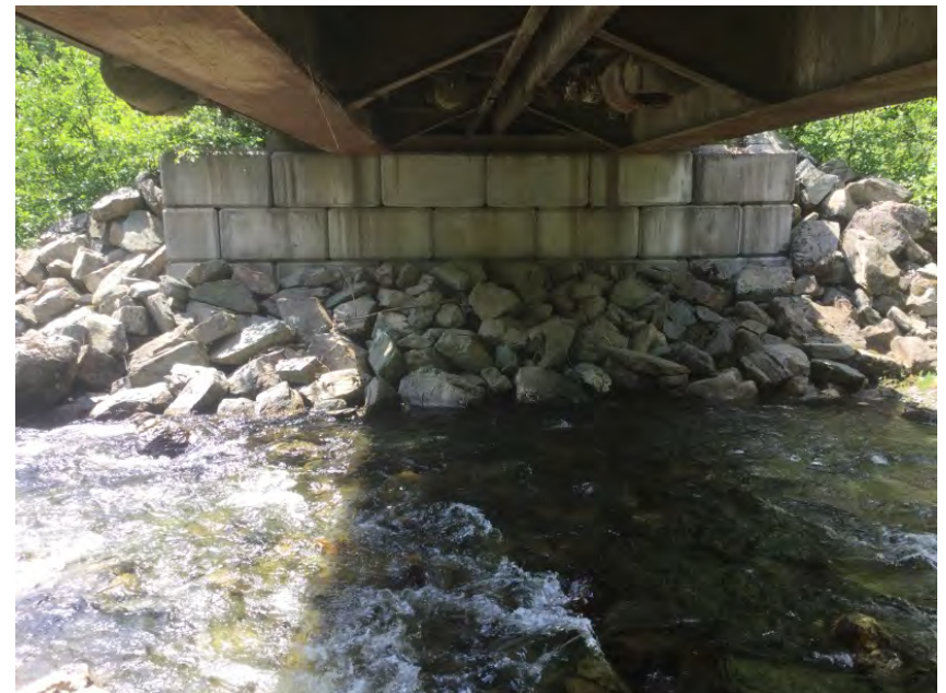
Right Bank Abutment when facing downstream
