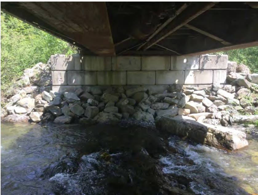
Left Bank Abutment when facing downstream
